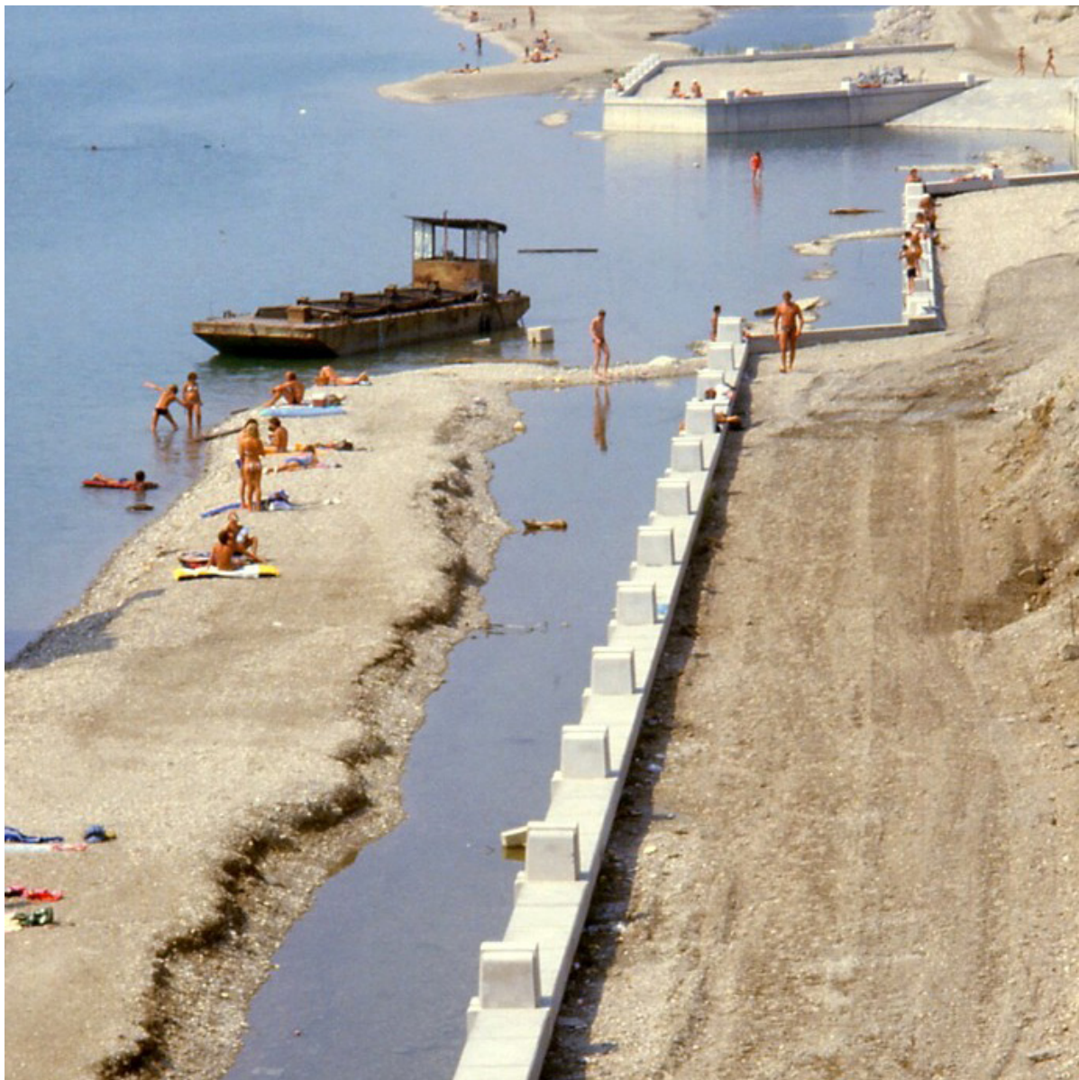
Image: Construction of Donauinsel, Vienna, 20 July 1983. Photograph: © TARS631, via Wikimedia Commons (attribution-only licence).
